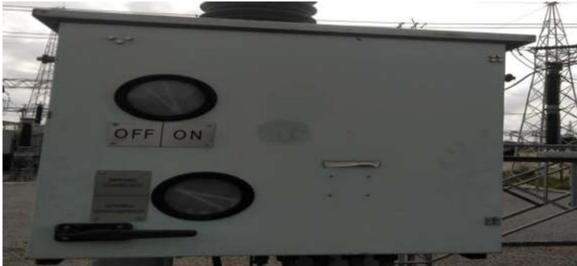
Fig: operating mechanism for breaker operation
