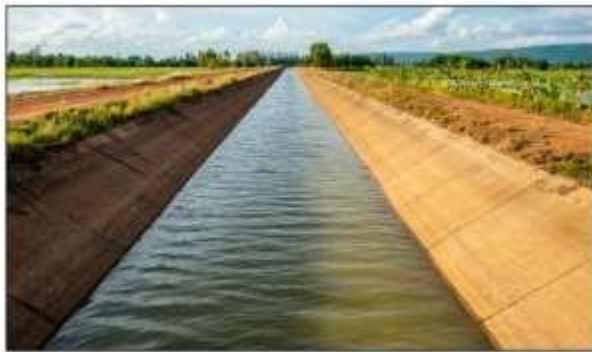
Figure: Irrigation canal
