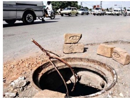
Figure .2: Opened Manhole
