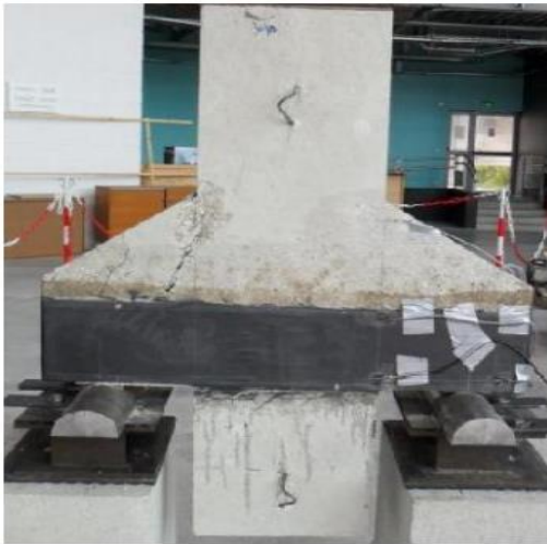
b) CB3u : Compression failure
