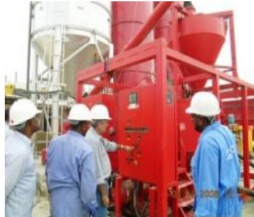
Figure 7: Insite slurry preparation
