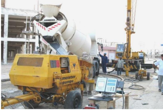
Figure 2: Delivery of cavity filling mix
