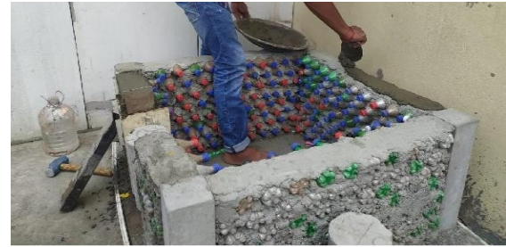
Fig 11. Construction of pet plastic bottle room
