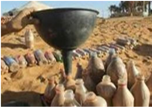
Fig 8. Filling the bottles with sand
