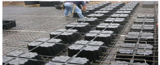
Fig 3. U-Boot technology in slabs
