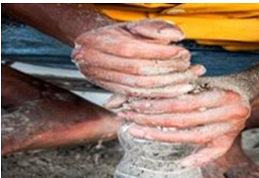
Fig 9. Compacting the bottles
