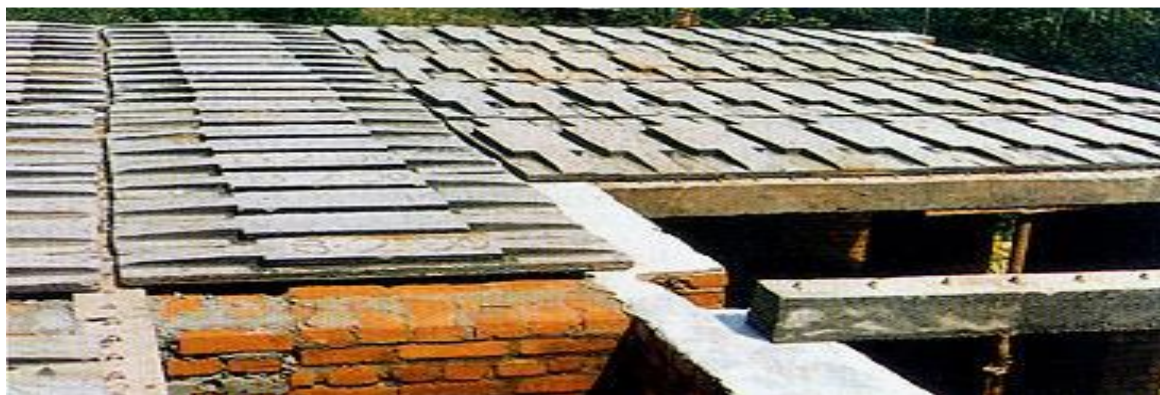
Fig. 3 R.C. Planks laid over partially precast joists
