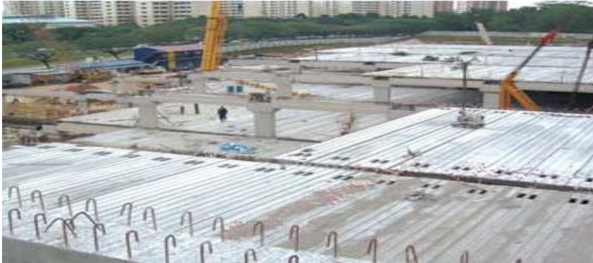
R.C. Planks laid over partially precast joists
